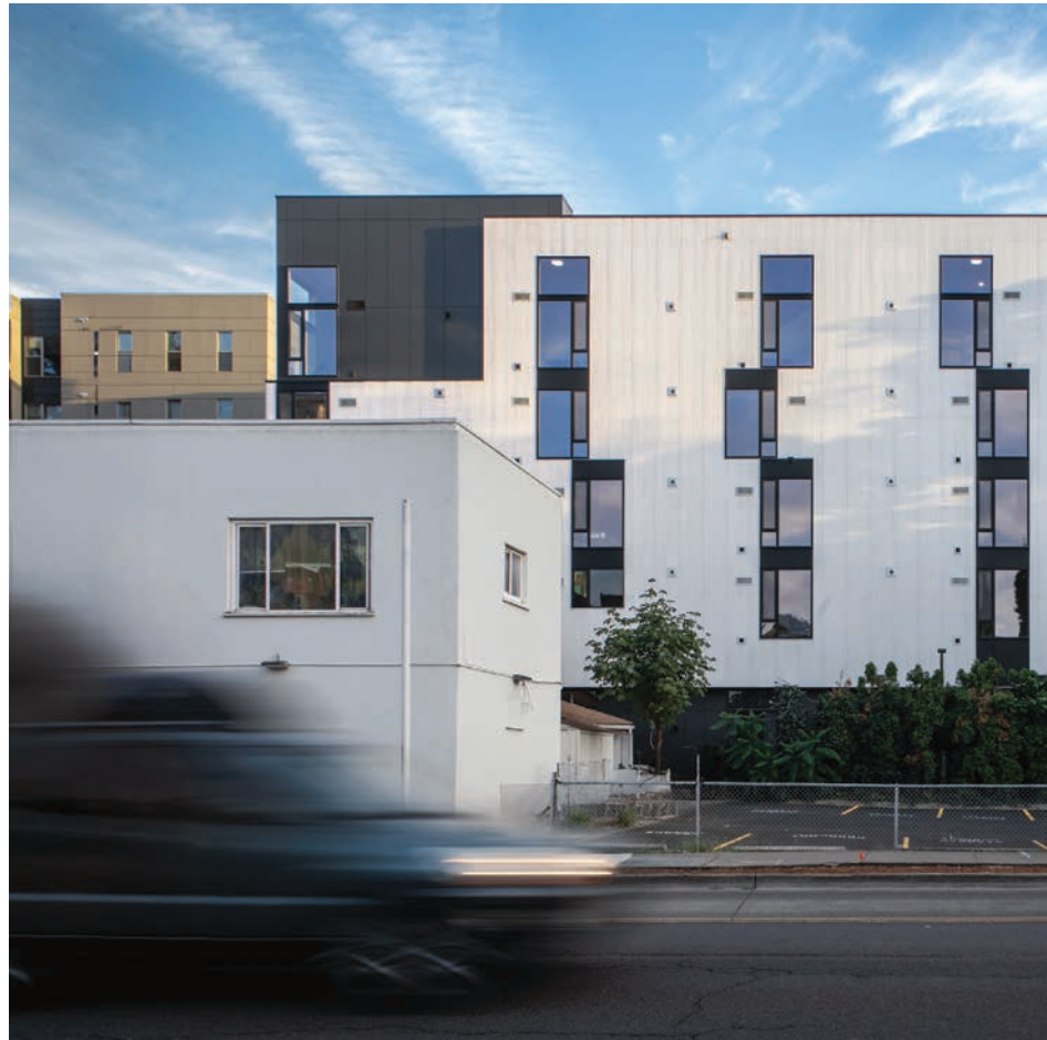
Ferry Street Flats' push-pull facade alternates metal cladding and black fiber-cement panels.
